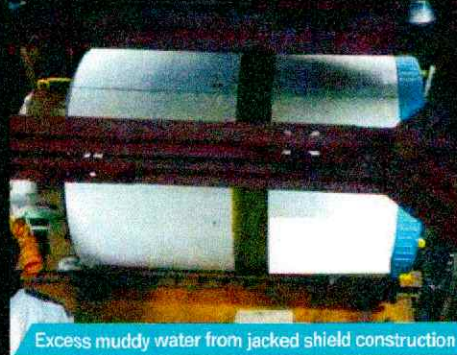
Excess muddy water from jacked shield construction
