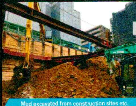
Mud excavated from construction sites etc.
