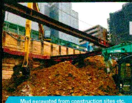
Mud excavated from construction sites etc.
